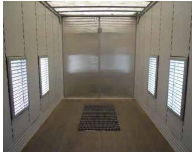
Floor Breather vent w/ Wall mounted intakes.
